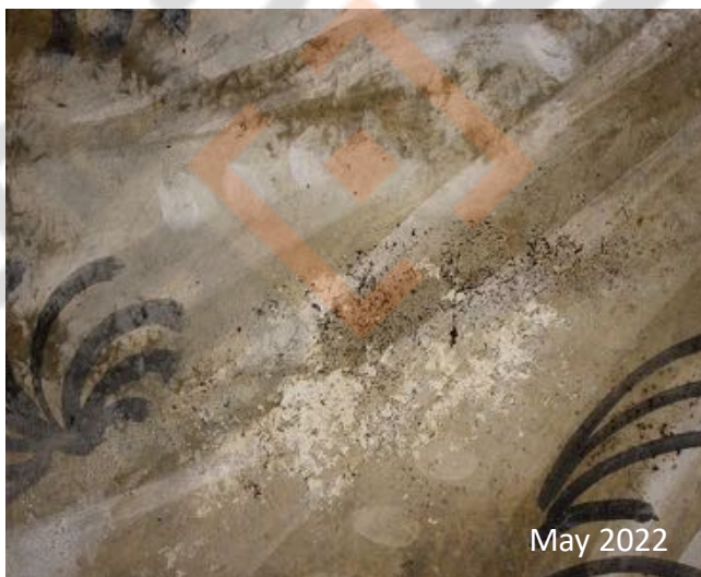
Figure 2a and 2b. Area of microbiological growth and salt efflorescence in incident (left) and raking light (right) on the east face of the vault on the west arm.
