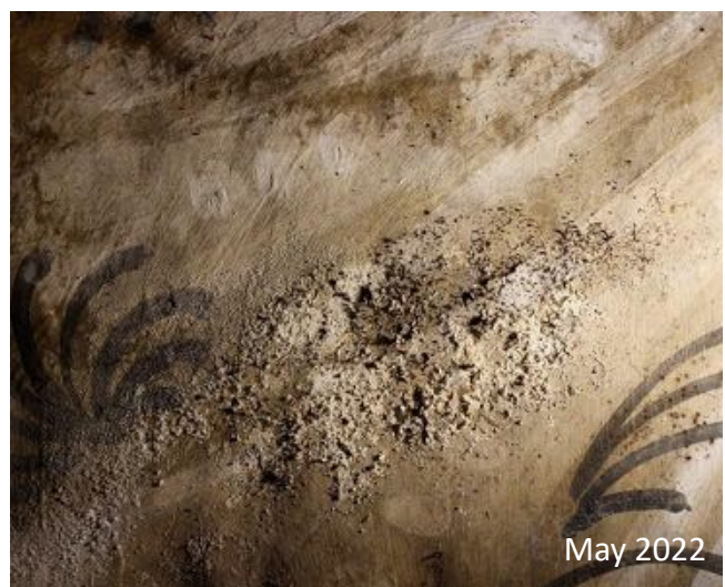
Figure 2a and 2b. Area of microbiological growth and salt efflorescence in incident (left) and raking light (right) on the east face of the vault on the west arm.
