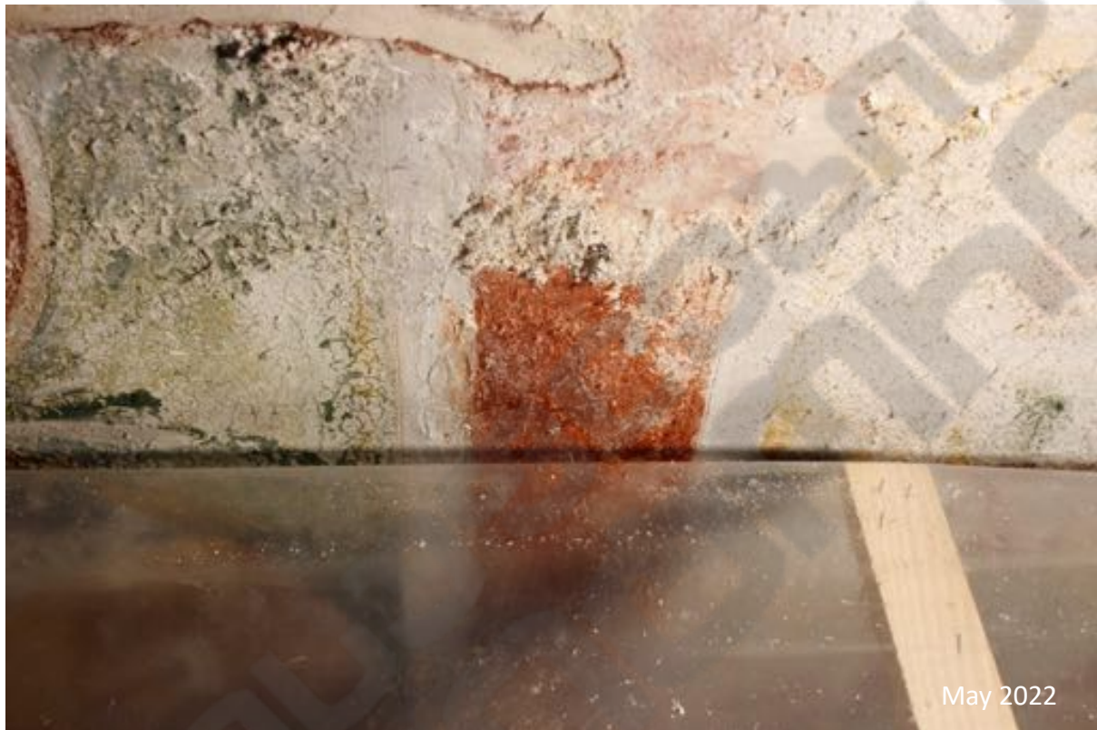
Figure 1 Active deterioration is apparent with widespread presence of crystallised salts on the surfaces of the paintings and ongoing paint loss, seen here on 2 May 2022 with newly accumulated paint fragments on the plastic sheeting.
